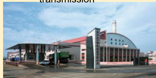
Hankou WTE facility
