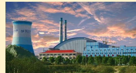
Wuchang WTE facility
