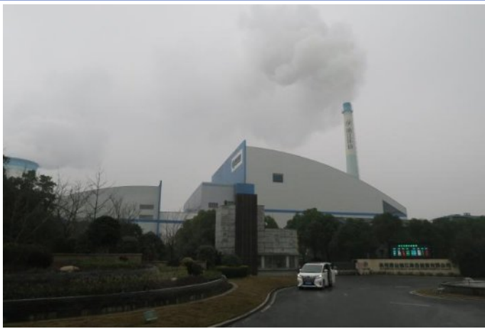
Source: CLSA; Note: Pictures taken by CLSA on 19 Jan 2017
